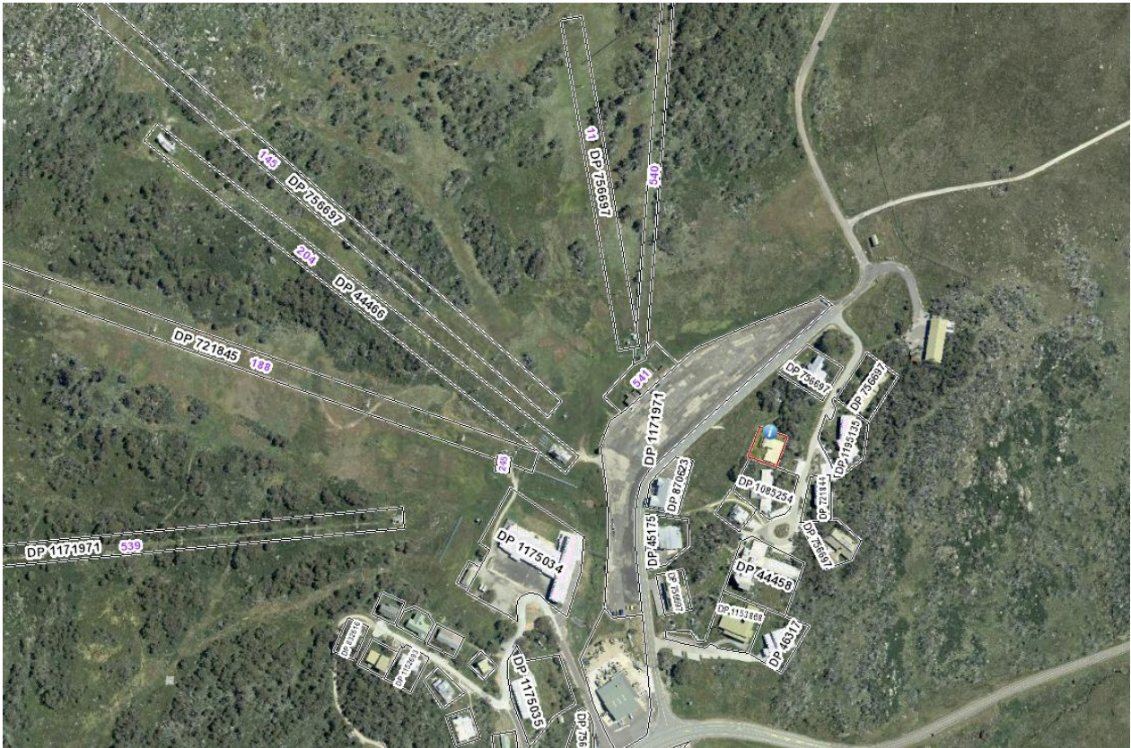
Figure 1: Context of the site within the locality
