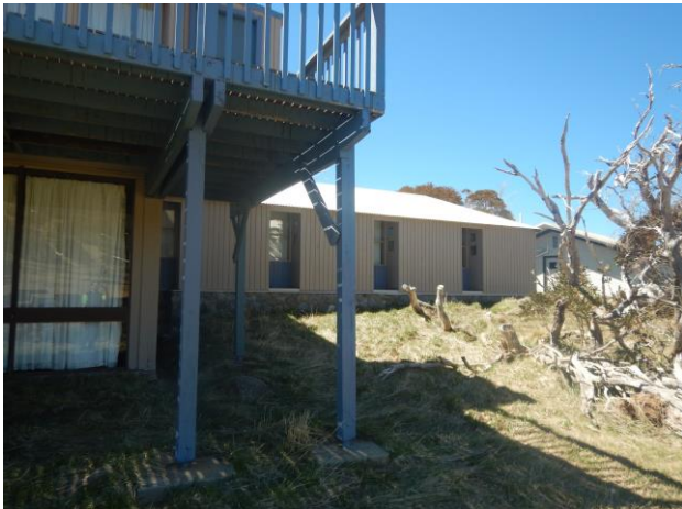
Figure 9: Photo of the western elevation of the lodge
